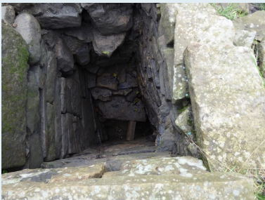
The 'shaft' in the pond bank.
